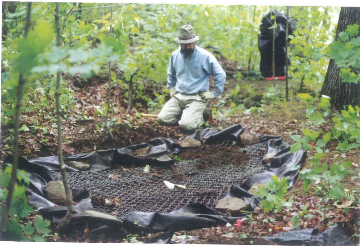
Fig. 4. To stabilize the pit, geotextile was placed as lining, then backdirt to fill, then chain link fencing with extra geotextile folded over its edge. Lindner looks on before backdirt is shoveled on top. Trowel in the pit points roughly north. Photo taken May 25, 2001.
